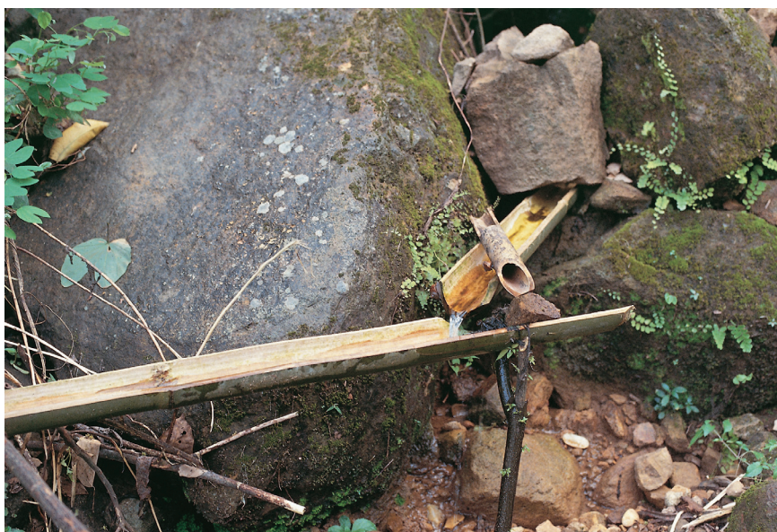
In India's north-east, bamboo pipelines are commonly used to transport water to be used for drinking or for irrigating fields
