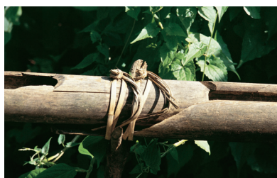
In India's north-east, bamboo pipelines are commonly used to transport water to be used for drinking or for irrigating fields
